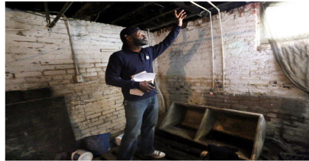
Akbar Tyler, an inspector with Environmental Health Watch, visits homes in Cleveland to check for mold, lead paint, standing water, roaches, animal droppings—anything that would be an asthma trigger or health hazard. The BUILD grant will help that organization, along with the Cleveland Department of Public Health and the MetroHealth System, to continue this work in three Cleveland neighborhoods. (Lynn Ischay, The Plain Dealer)
