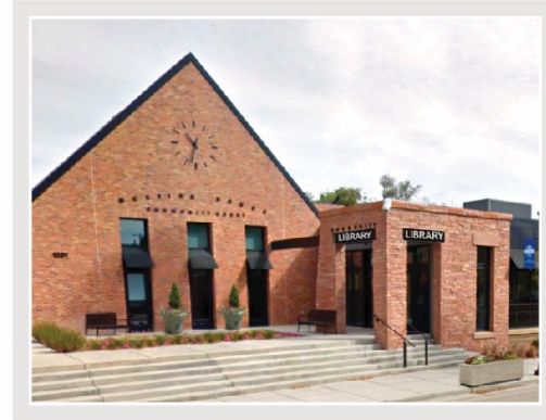
PHOTO 2 LIBRARY WITH SMALL-SCALE ENTRANCE IMPROVEMENTS
