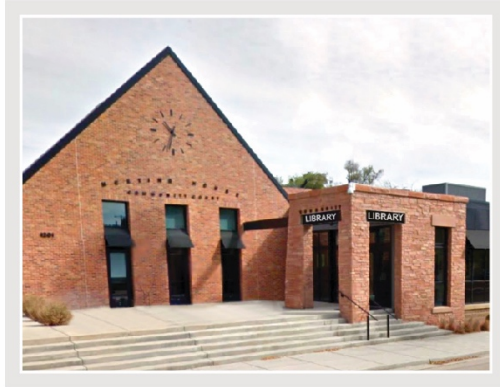
PHOTO 1 LIBRARY WITHOUT ENTRANCE IMPROVEMENTS
